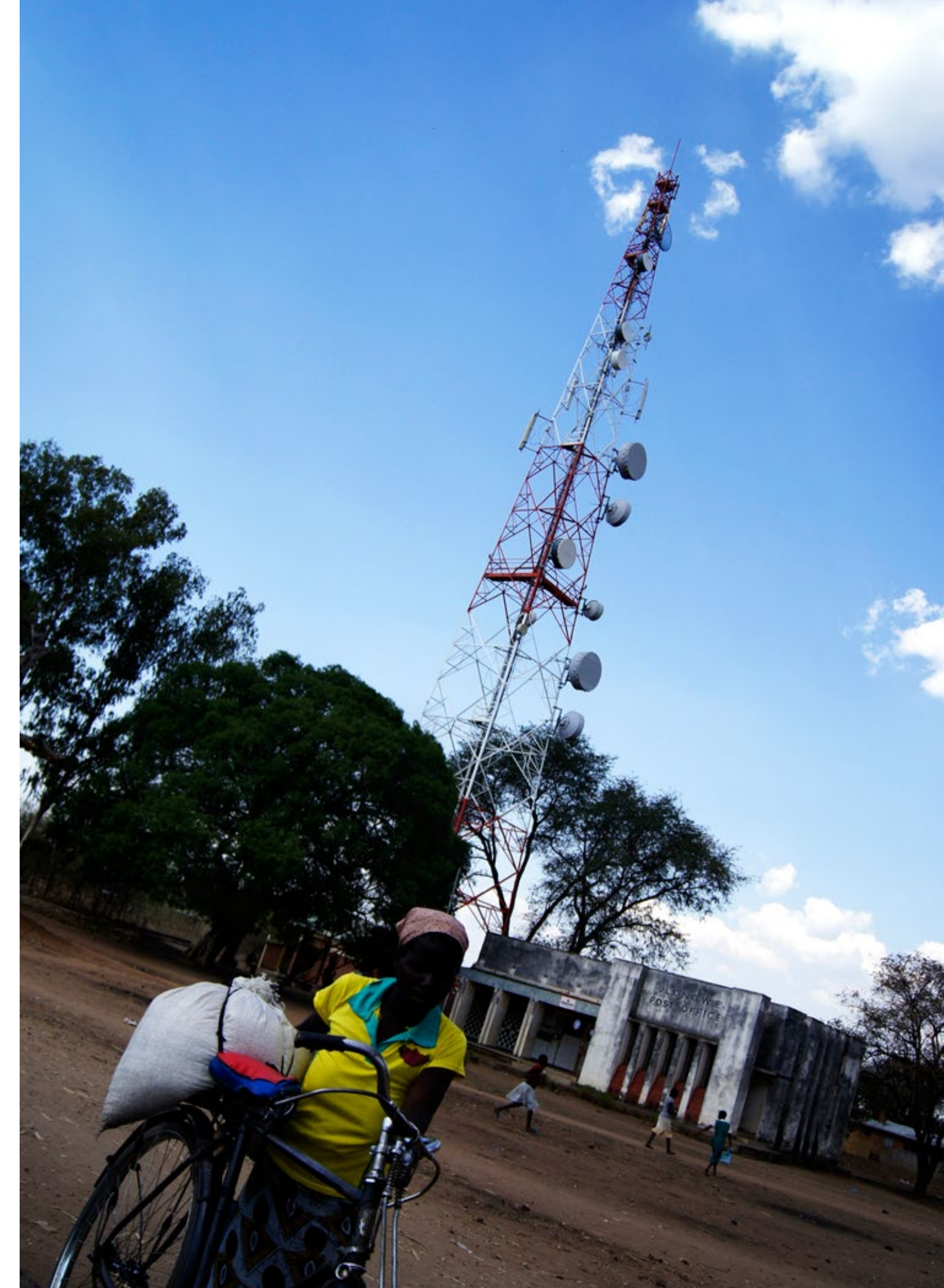
A recently-built mobile network tower next to a dilapidated post office in rural Ulongwe, Malawi.
